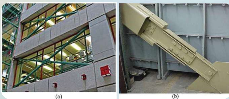
Photo 1. Pall friction damper: (a) structural application and (b) connection of damper to structure. (Heysami 2015)
