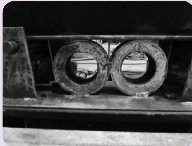
Photo 6. Infilled-pipe damper
