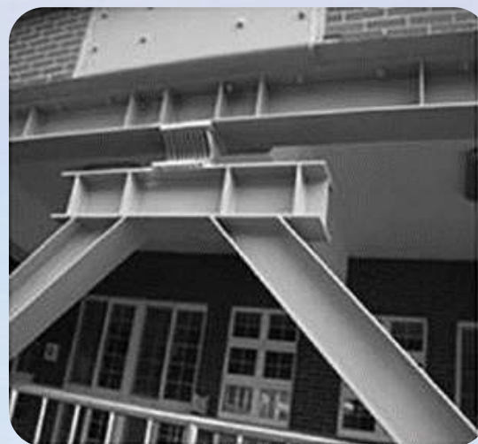
Photo 1. Metallic dampers installed in a building
