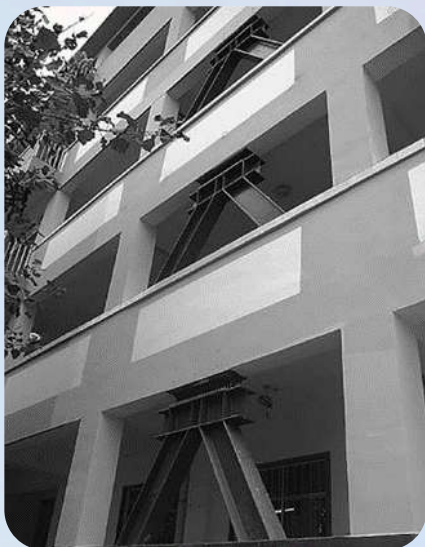
Photo 1. Metallic dampers installed in a building
