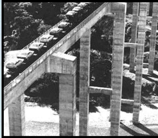
PHOTO 1. APPLICATION OF SELF-CENTERING SYSTEM ON THE RANGITIKEI RAILWAY BRIDGE, NEW ZEALAND. (CHRISTOPOULOS ET AL. 2002.)
